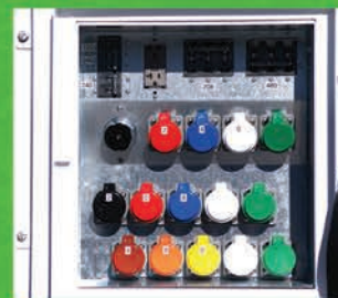
Single-Phase (110/240V) and Three-Phase (208/240/480V) Receptacle Outlets
