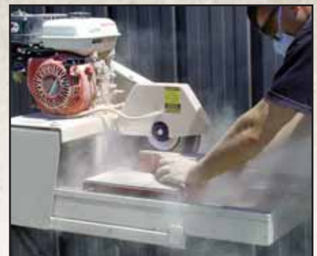
WITHOUT DUST CONTROL
