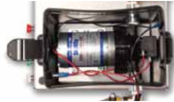
12V Booster Pump is protected in an all-weather box.
