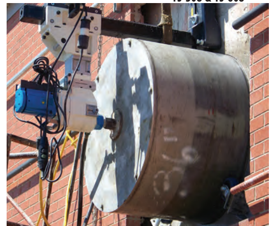
TS-603 drilling with a 36" bit at a water treatment plant.
