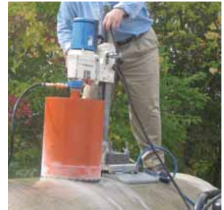
Twin Pipe Pad for drilling concrete pipes
